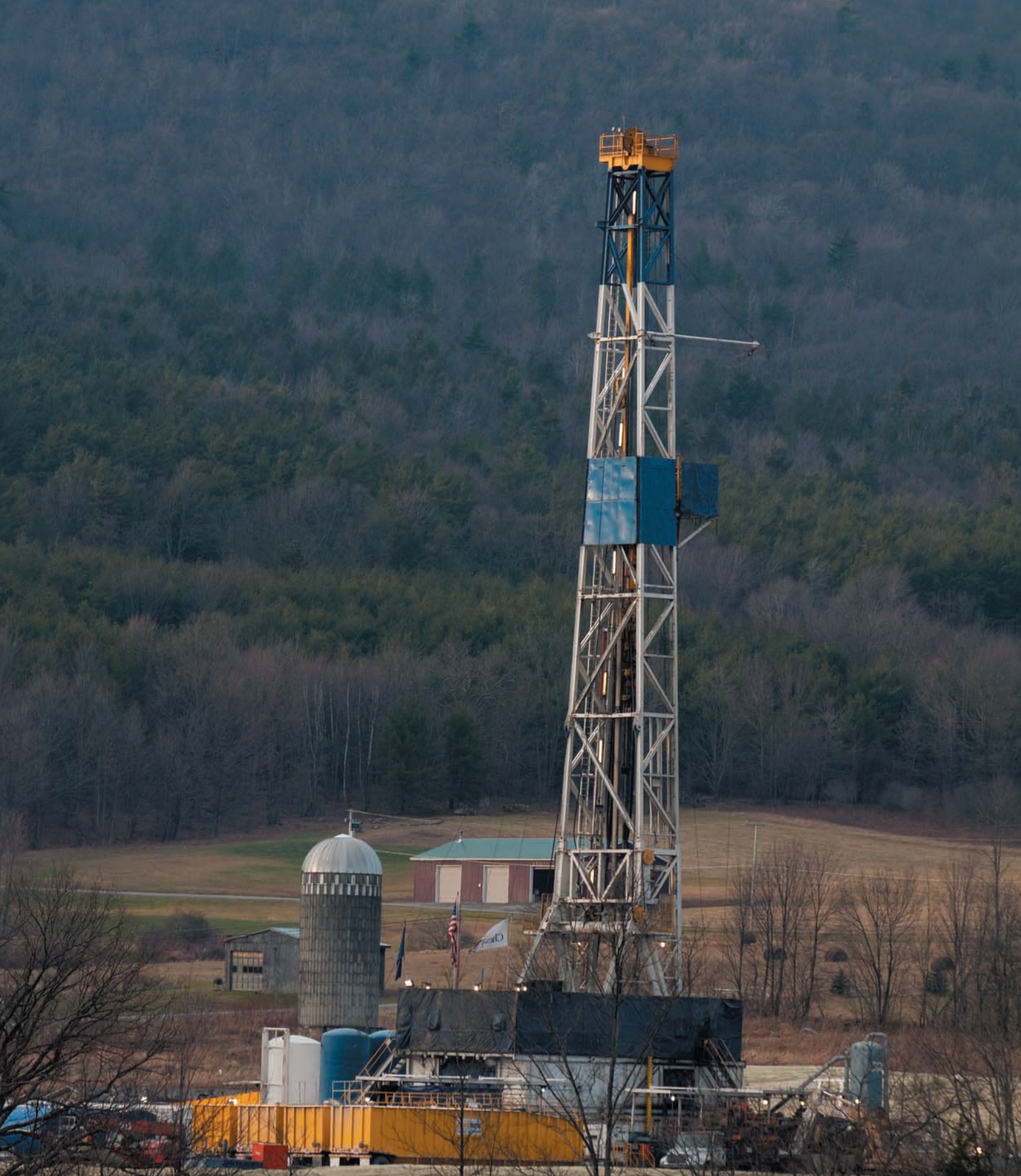
A hydraulic fracturing site like this one near Canton, Pennsylvania, can contain many features that are seen prominently here including a concrete pad, a drilling rig, and many storage containers. (Les Stone/Corbis)
